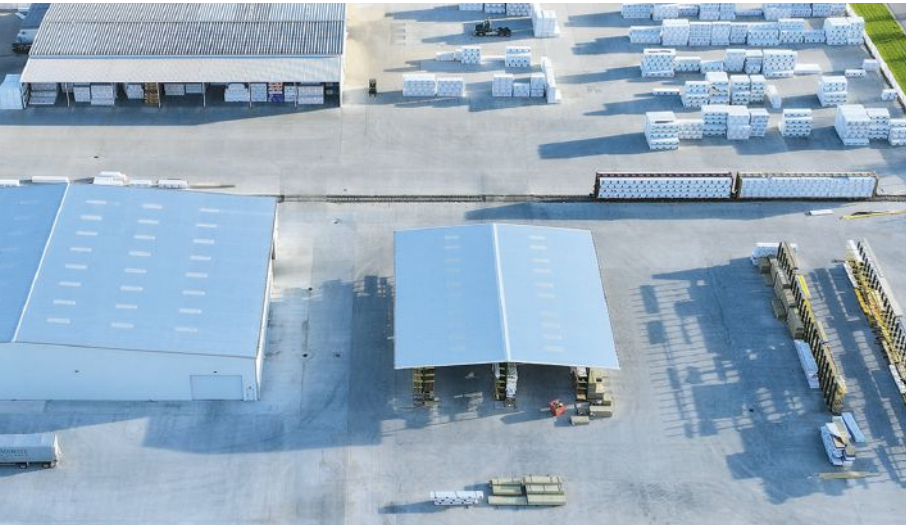
This facility, constructed for Sprenger Midwest Wholesale Lumber in Moorhead, MN by CT Darnell, consists of multiple components, including a 6,000-sq. ft. three-sided bulk storage shed, a 32,000-sq. ft. warehouse building, and a 11,500-sq. ft. double-aisle cantilever rack-supported drive-thru building.
