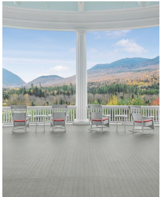
ACRE Porch Flooring | Mt. Washington, NH
