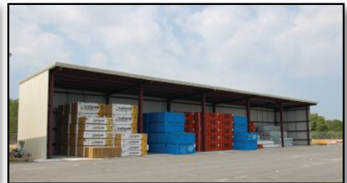
Bulk Storage Sheds
