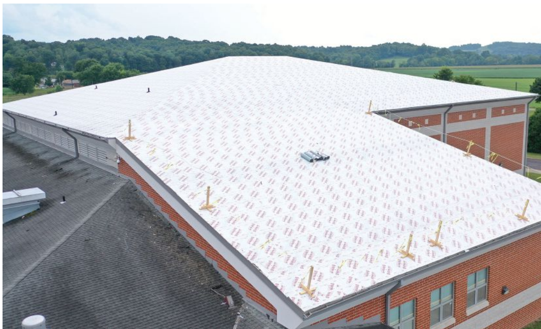
MFM Ultra HT Wind & Water Seal is a 45-mil, self-adhering roofing underlayment composed of a white, non-slip, cross-laminated polymer film, laminated to a high-temp rubberized aggressive asphalt adhesive. According to MFM, it can be used under shingle, tile, shake, and metal roofing systems. It bonds to the substrate and seals around fasteners to limit damage caused by water penetration or leaks.
