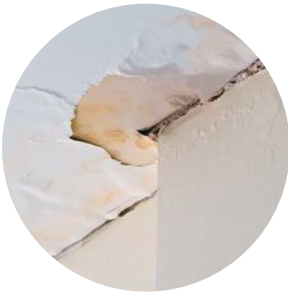
Damage caused by conventional boot failure
