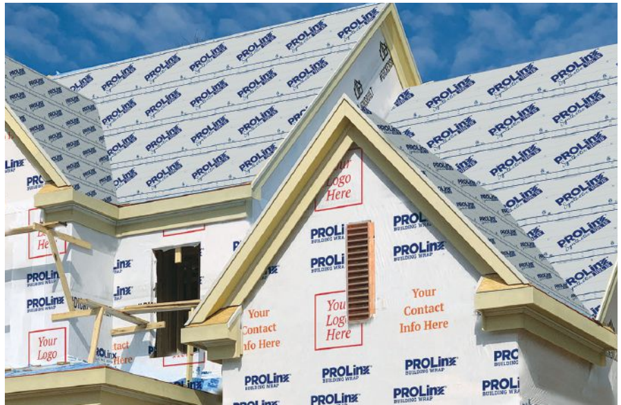
ABOVE: PROLinX Select Building Wrap from BlueLinX is a woven fabric weather barrier that can be customized with a builder’s logo and contact information. According to the manufacturer, it provides exceptional strength and durability at a low weight, and it is available with some of the smallest minimums in the industry.
