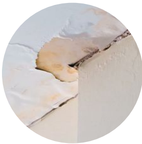
Damage caused by conventional boot failure
