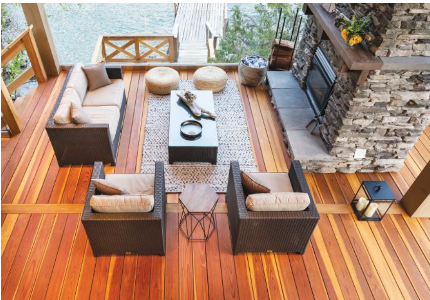
LEFT: Humboldt Sawmill is working on new redwood decking products treated with an in-cylinder fire retardant treated formulation to achieve Class A flame spread. These products are being tested in limited markets where wildfire potential is elevated and/or where local building codes have begun to mandate Class A decking products.
