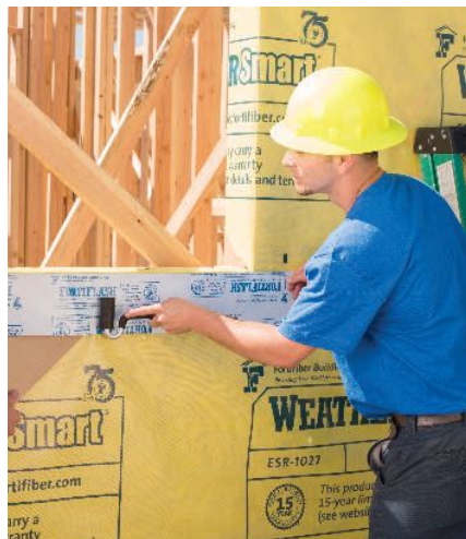
RIGHT: According to Henry, its WeatherSmart Housewrap protects against water and air intrusion from the outside while allowing moisture to escape from the inside. It features an advanced polymer technology, is suitable for use in any climate, and can be used behind most exterior claddings including fiber cement, brick, vinyl and wood siding.
