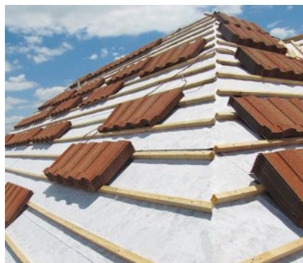
ABOVE: In 2019, MFM introduced Premium HT Tile & Metal Underlayment for use under tile and metal roofing systems. According to MFM, the new product features a polyester top surface to hold stacked tiles in place, offers great traction for the roofing contractor, and is rated to 250°F to withstand the extreme temperatures generated by metal roofing systems.
