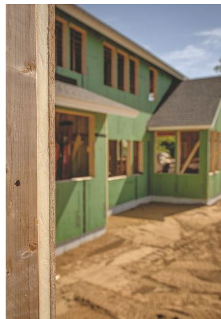
Huber Engineered Woods' ZIP System building enclosure products eliminate the need for loosely-applied water- and air-barriers such as housewrap in wall assemblies and felt in roof assemblies.
