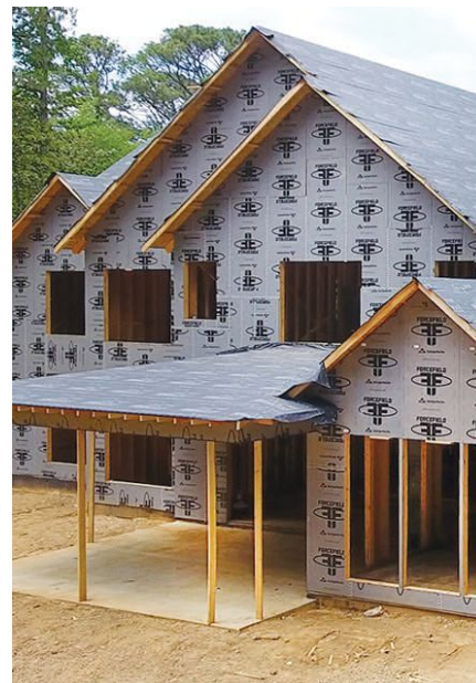
Georgia Pacific's ForceField Air & Water Barrier System is an integrated air and water barrier that, according to the manufacturer, eliminates the need for house wrap. The product also helps prevent air infiltration and exfiltration to create a more energy efficient home and meet newer air exchange requirements in the building codes.
