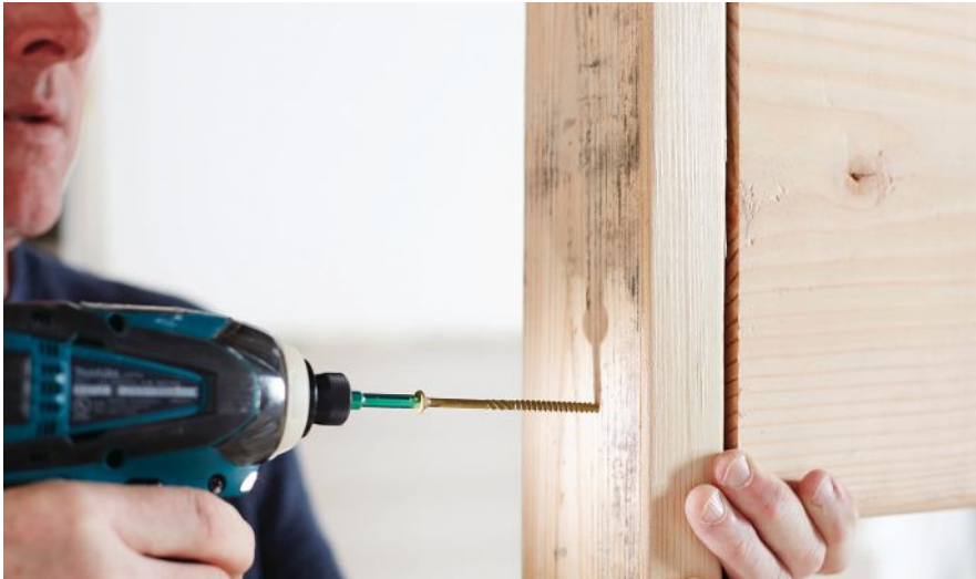
ABOVE: GRK will be introducing improvements to its R4 multipurpose framing and decking screw in December. The new screws will have several changes designed to increase efficiency, including tips that engage more quickly, a better fit between the head and bit, and an improved thread design.
