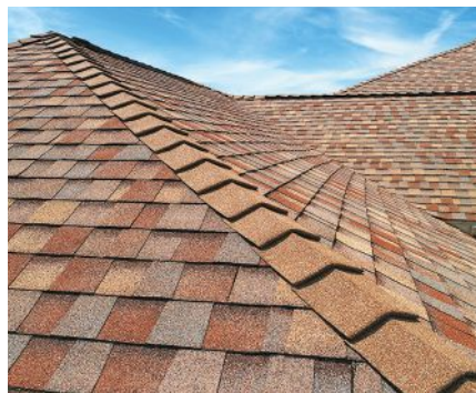
RIGHT: TAMKO’s new Heritage® Designer Ridge is a high profile ridge product that adds a look of polished sophistication to finish asphalt roofing projects with style. Constructed with SBS modified bitumen technology, two layers of asphalt shingles are laminated together to produce the high-definition appearance of added dimension.
