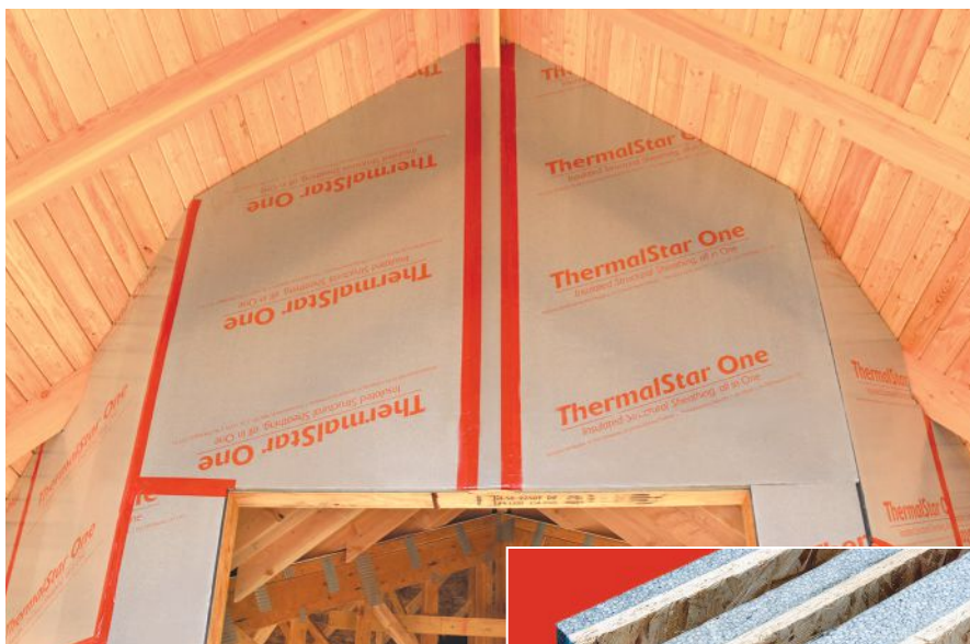
Universal Forest Products' ThermalStar One insulating structural sheathing combines four layers in one application that according to the manufacturer provides a strong, stiff, nailable structural layer with segment leading shear value, graphite enhanced rigid insulation in three thicknesses/R-Values, and an integral taped WRB/air barrier layer.
